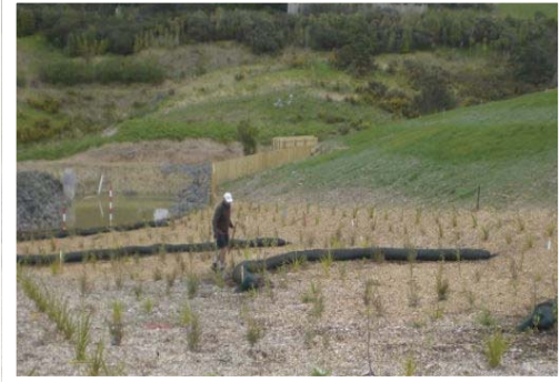
300mm Siltstop used to control overland flow velocity thereby removing sediment and other debris by sedimentation and filtration
