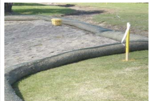
300mm Siltstop used as cost-effective silt fencing for construction projects (Manukau, NZ)
