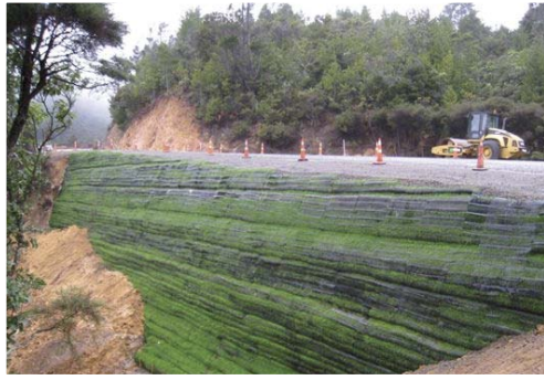
300mm Siltstop used for road support (State Highway 26, New Zealand).
